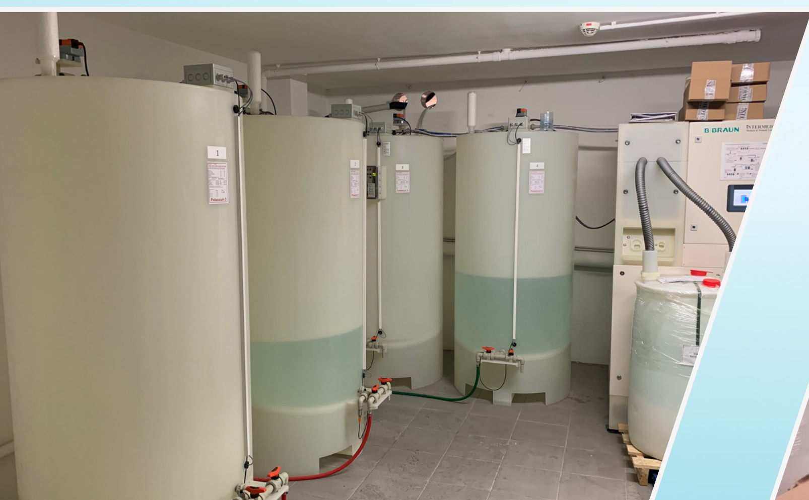
Installation ECOMix Revolution Saint Pierre
